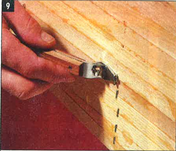
PULL THE STAPLES out when all the strips are in place and the glue is dry. A bottle opener with the tip ground or filed flat is the perfect tool.
